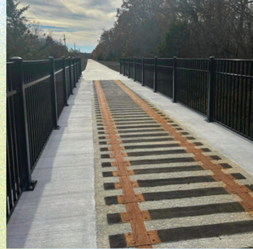
The Chadwick Flyer Trail will ultimately connect southeast Springfield in Greene County to downtown Ozark in Christian County.
