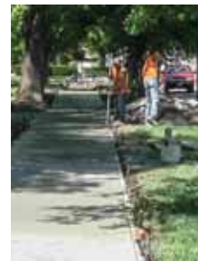
Sidewalk construction at Benton Avenue and Calhoun Street.
