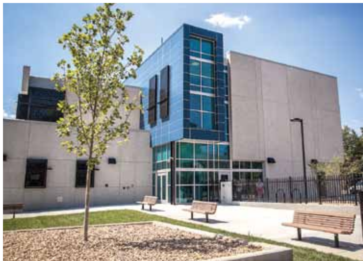
The Springfield-Greene County Public Safety Center opened in 2012.
