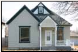
Neighborhood Stabilization Program Rehab Property of Urban Neighborhoods Alliance
