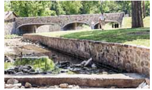
Fassnight Park’s completed Waterway/Stormwater Improvement Project.
