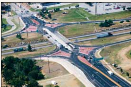
Kansas Expressway and I-44 Diverging Diamond Interchange
