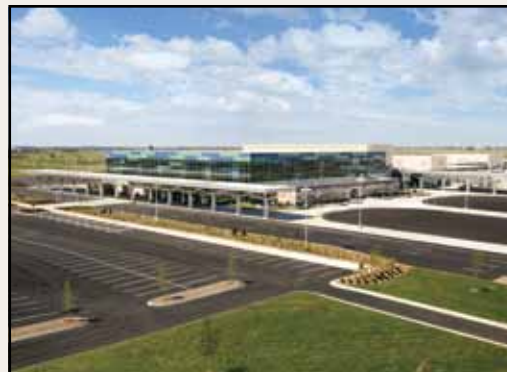
Springfield-Branson National Airport Terminal
